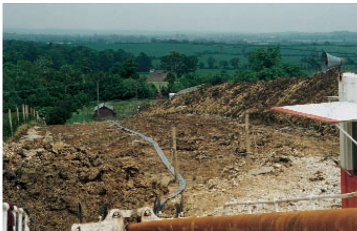
View of the drilling route to the exit point 30 m below.
