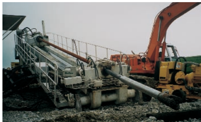
Stockton 100 t rig fitted with DigiTrak guidance system.
