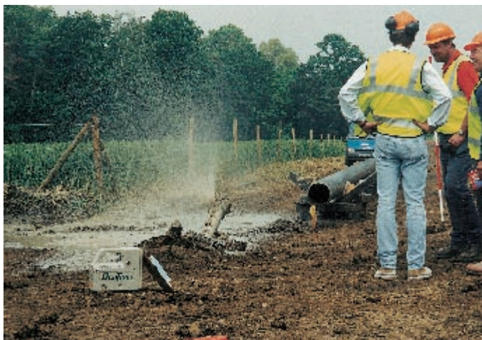
A precise exit completes the pilot bore.
