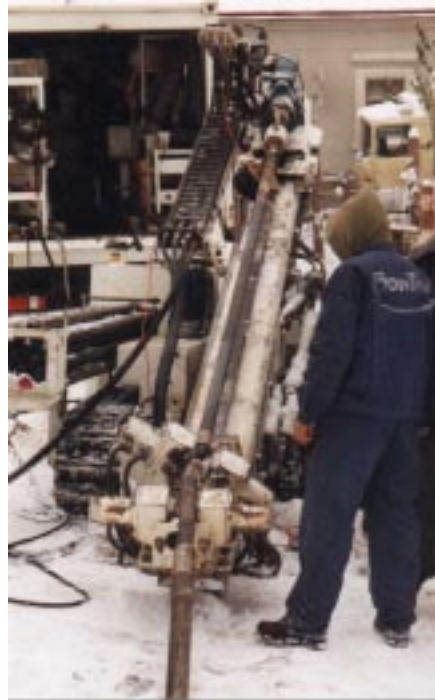
Wiring Cable Transmitter from top of drill string to drill housing in lower section.
