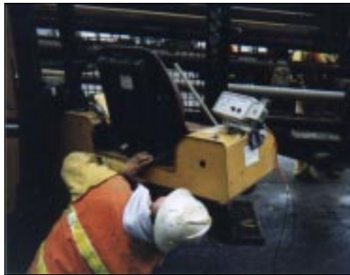
Drill operator checking power supply ground connections for Cable Transmitter System.
