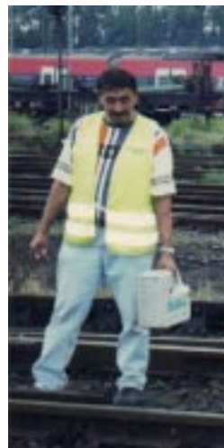
DigiTrak operator verifying borepath.
