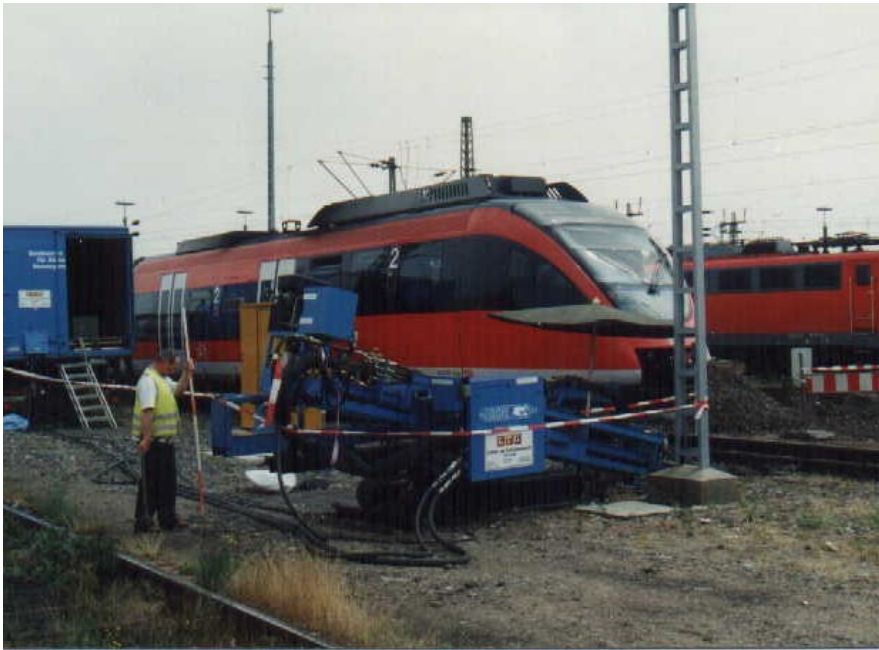
LTG setting up Tracto-Technik Grundodrill rig at edge of tracks
